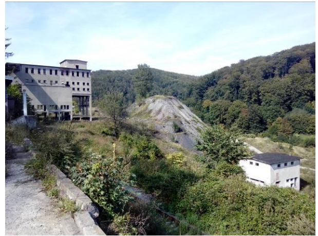
Figure 9. Dumps, ground heavily affected
