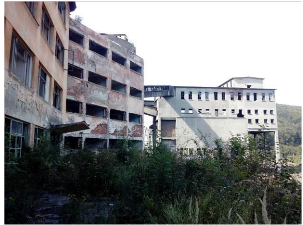
Figure 6. The offices and coal sorting building
