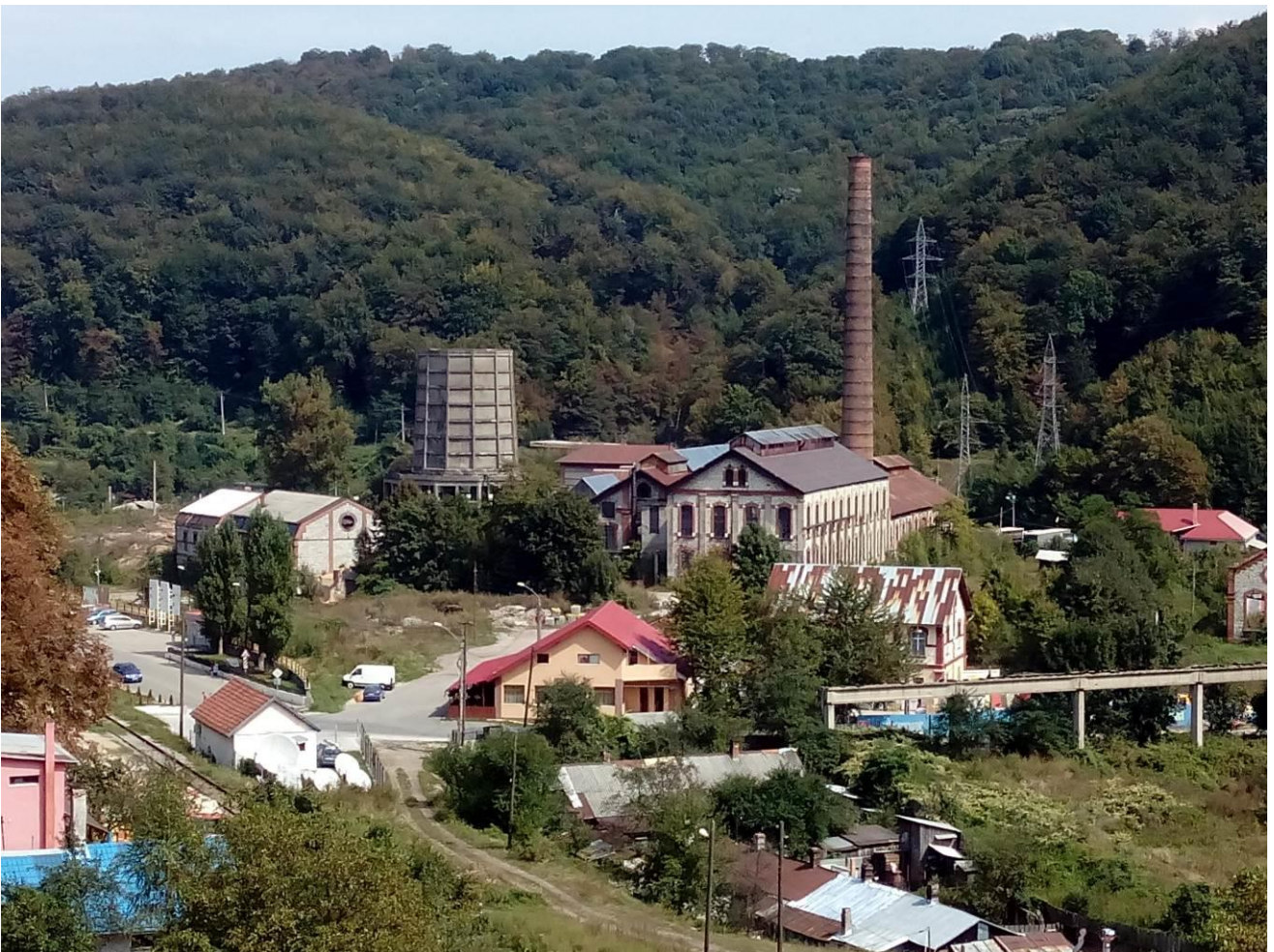
Figure 10. Overview of the power station
